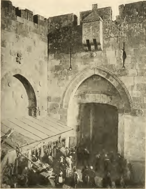
THE GATE, JOPPA
